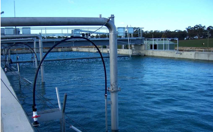
Picture - Mulwala Sewerage Treatment Works – Completed November, 2008
